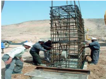
Fig. 6. Bar cage placement, guide frame.
