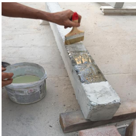
Fig. 4. Applying epoxy resin to concrete surface.
