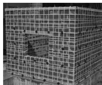
Fig 21. Application of Polypropylene bands.
