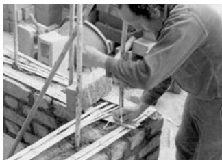
Fig. 16. Cane or timber internal reinforcement.
