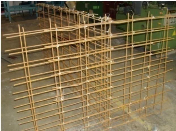
Fig. 5. Skeleton of wall-slab consist BRC-7.
