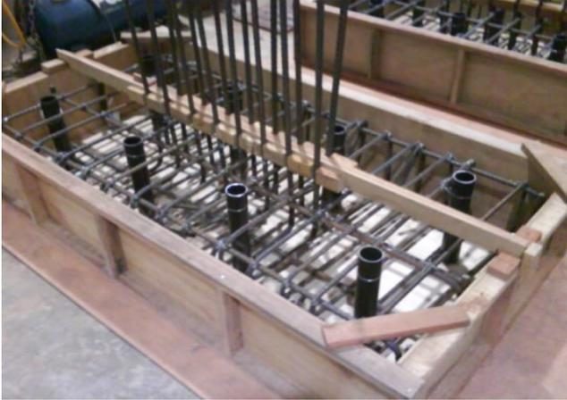
Fig. 4. Preparation of foundation beam cage.
