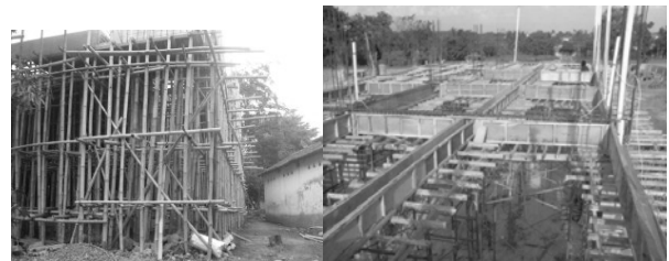
Fig. 3. Conventional system using wood for formwork and scaffolding.
