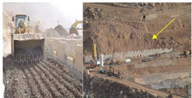
Fig. 5. Embankment operation (a), General view of structure (b).
