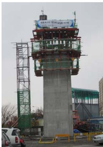
Fig. 14. Completed concrete pylon with tapered section.
