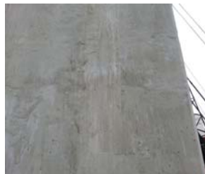
Fig. 13(b). Surface of concrete (surface wave velocity > 1100 m/s).
