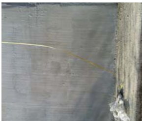
Fig. 13(a). Surface of concrete (surface wave velocity < 1100 m/s).
