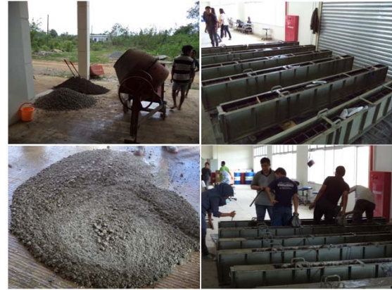
Fig. 3. Test preparation materials and casting beams.
