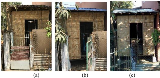
Fig. 3. Types of Bamboo House in Tropical Region, Myanmar. (a) Bamboo House with Dani roof; (b) Bamboo House with GI Roof; (c) Bamboo House with Double Roof (Dani + GI).
