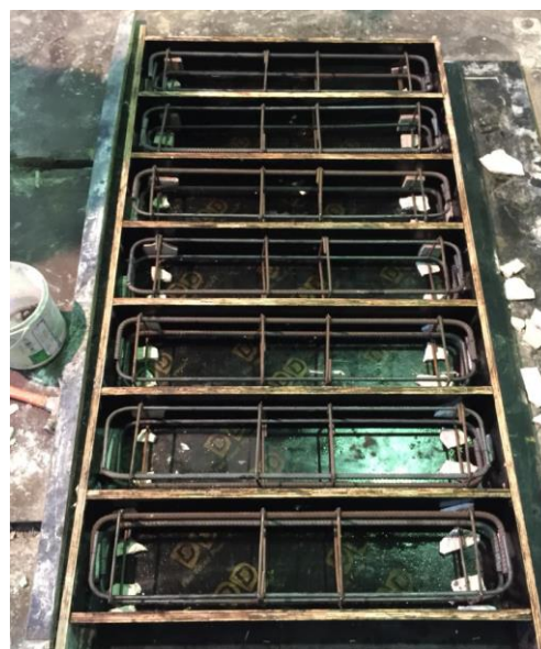
Fig. 3. Construction of RC beams
