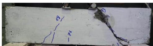
Fig. 8. Failure mode of beam 1-CON.
