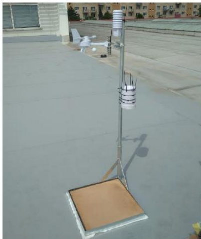
Fig. 2. The technical station for monitoring of humidity and temperature in roof deck and exterior.
