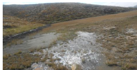
Fig. 2. Slope water seepage of Mengku dam.
