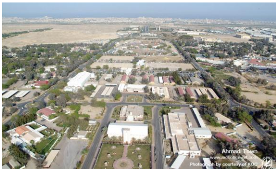
Fig. 2. Existing Ahmadi Township.
