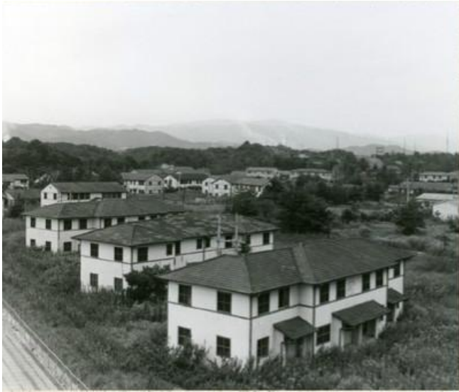
Fig. 4. Housing in kasugabaru base.
