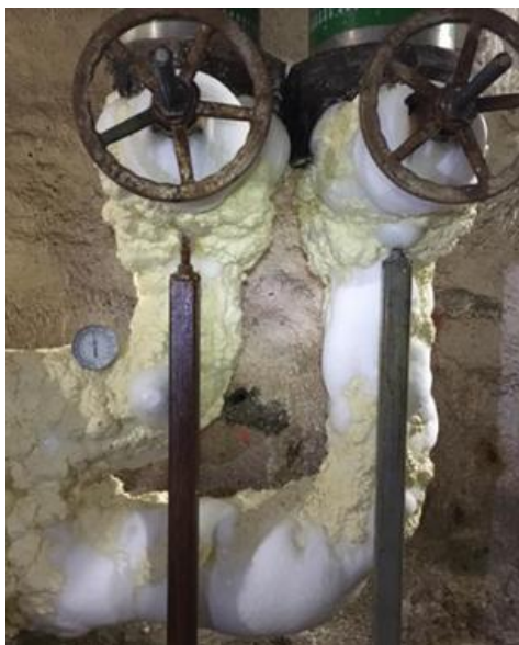
Fig. 1. Freezing of cryogenic insulation.
