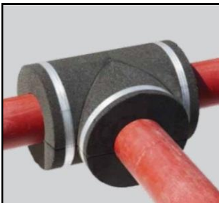
Fig. 5. Installation of tee insulation.
