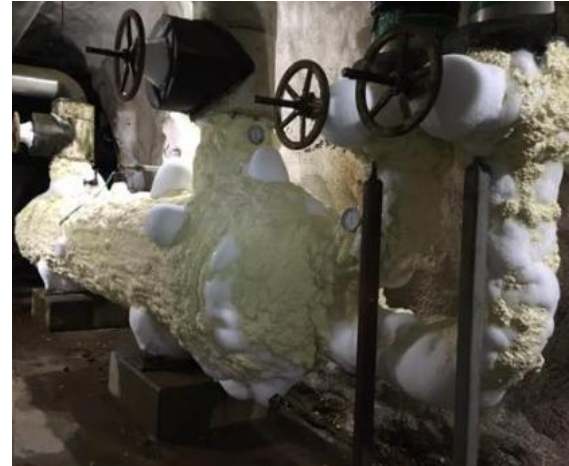
Fig. 2. Freezing of cryogenic insulation.
