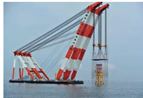
Fig. 1. Offshore support structure installation by crane lifting.
