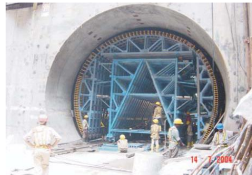
Fig. 5. View of tunnel of Delhi Metro Rail Corporation where fly ash has been used.
