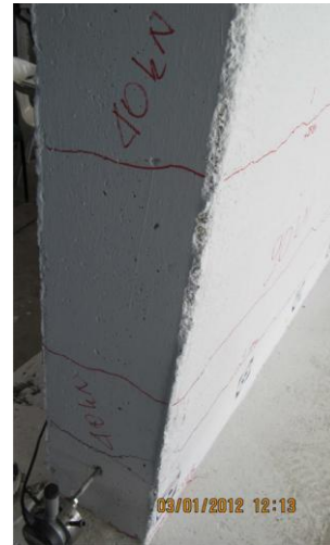
Fig. 8. Cracking patterns of SW1 at 40kN lateral load level.
