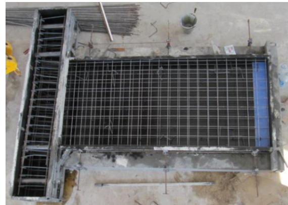
Fig. 5. Top view of the test specimen (SW1) in the construction stage.
