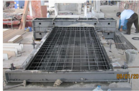
Fig. 4. Front view of the test specimen (SW1) in the construction stage.
