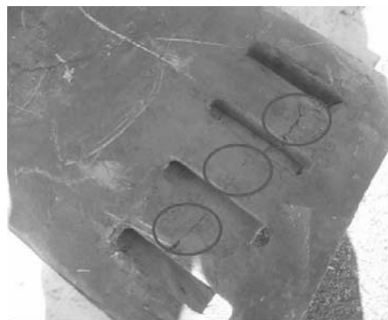
Fig. 4. Photo UHPC2.5 specimen cracks after 6-meter high free falling test
