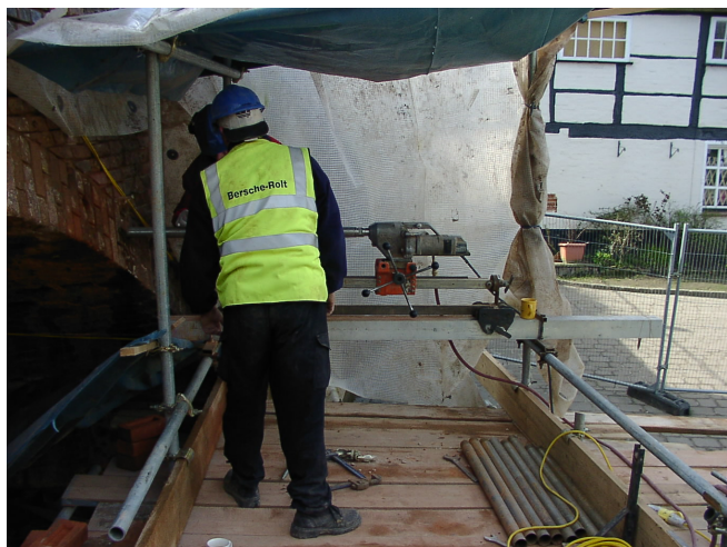
Fig. 2. Drilling the transverse holes in the arch barrel.
