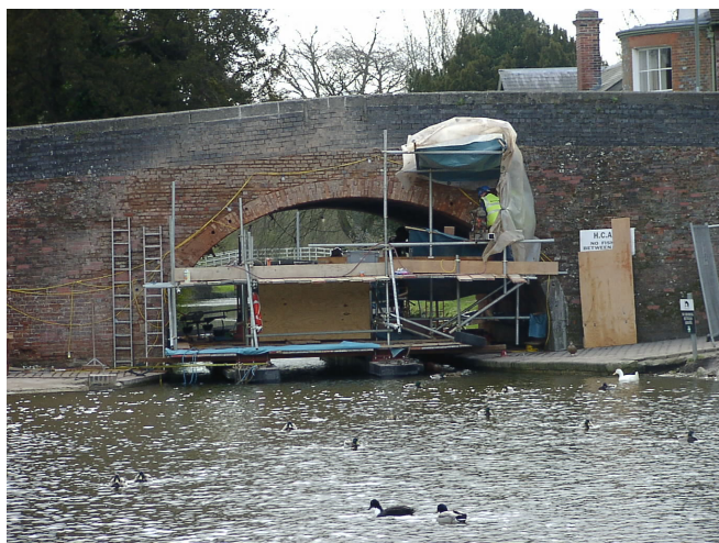
Fig. 1. Hungerford Canal Bridge showing the pontoons and working platform.
