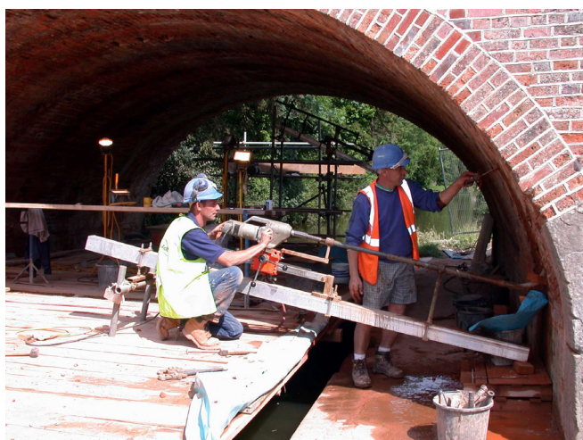
Fig. 3. Drilling the holes for the longitudinal reinforcement.
