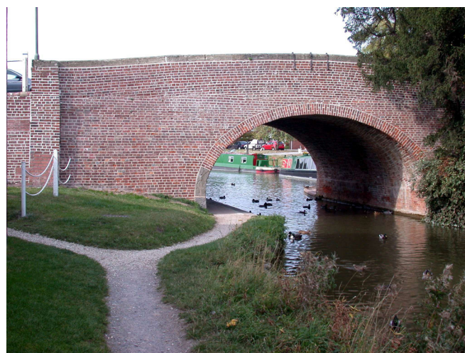
Fig. 5. A view of the successfully strengthened bridge.
