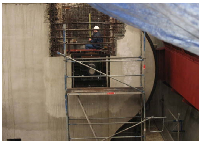
Fig. 4. Levelling measurement of the shaft axis – the last one – point D.
