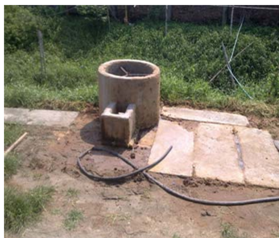
Fig. 1. Feed well of the digester
