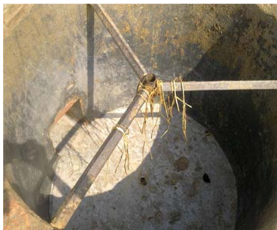
Fig. 4. Inside View of feed well digester
