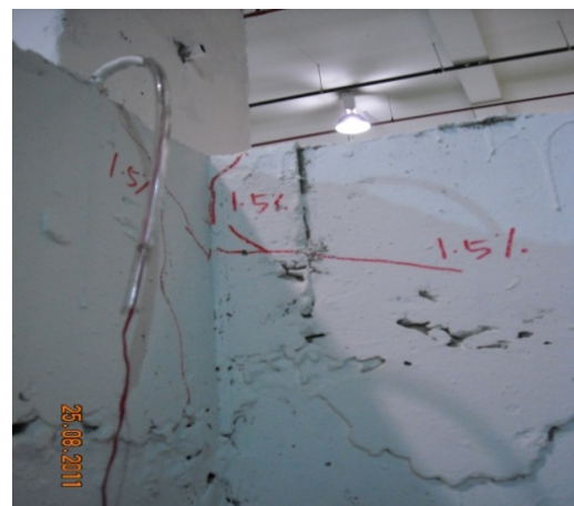
Fig. 9. Wider cracks were observed at +1.5\% drift.
