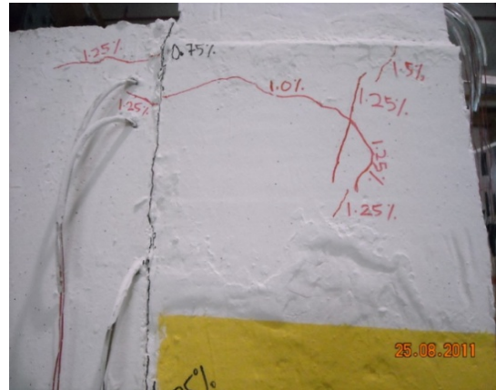
Fig. 8. Hairline cracks were observed at cast-in-situ beam-column joint located at upper part of the corbel.
